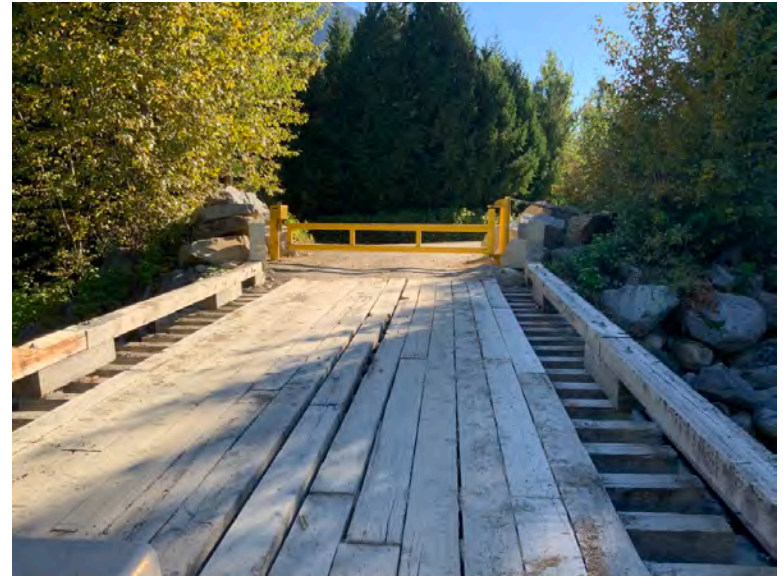
Approach from Right Bank when facing downstream
