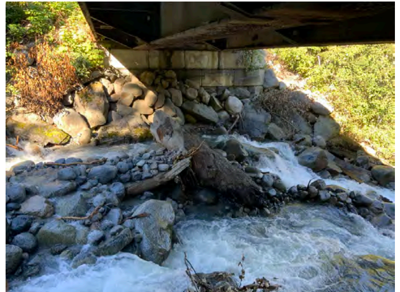
Left Bank Abutment when facing downstream
