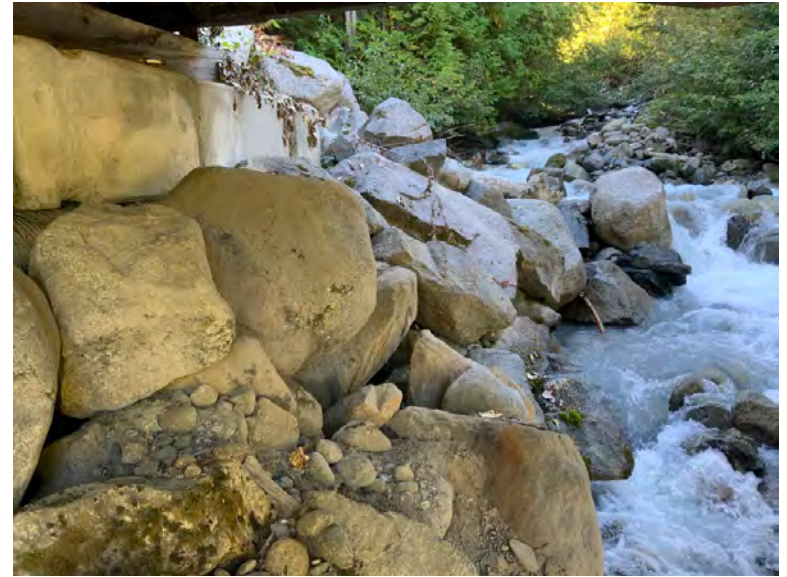
Right Bank Abutment when facing downstream
