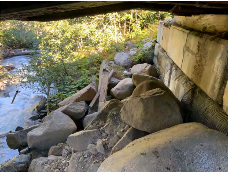
Right Bank Abutment when facing downstream
